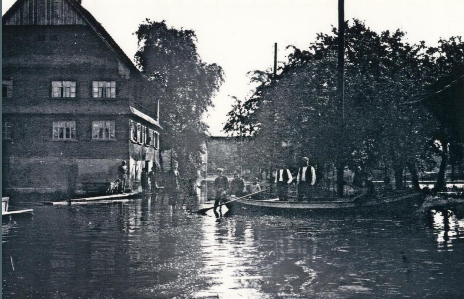
Flood in Lustenau
